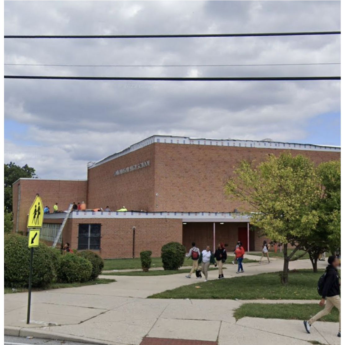
New roof being installed at Edmondson High
